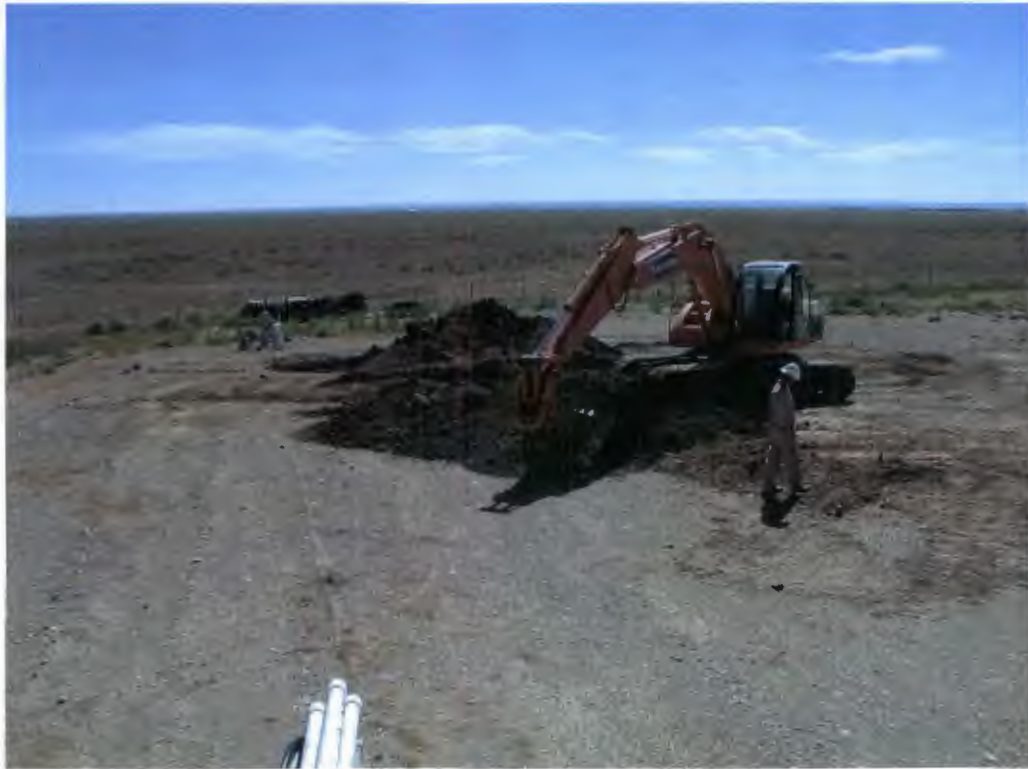
Excavating trench #3 in the former Pit #2 area.
