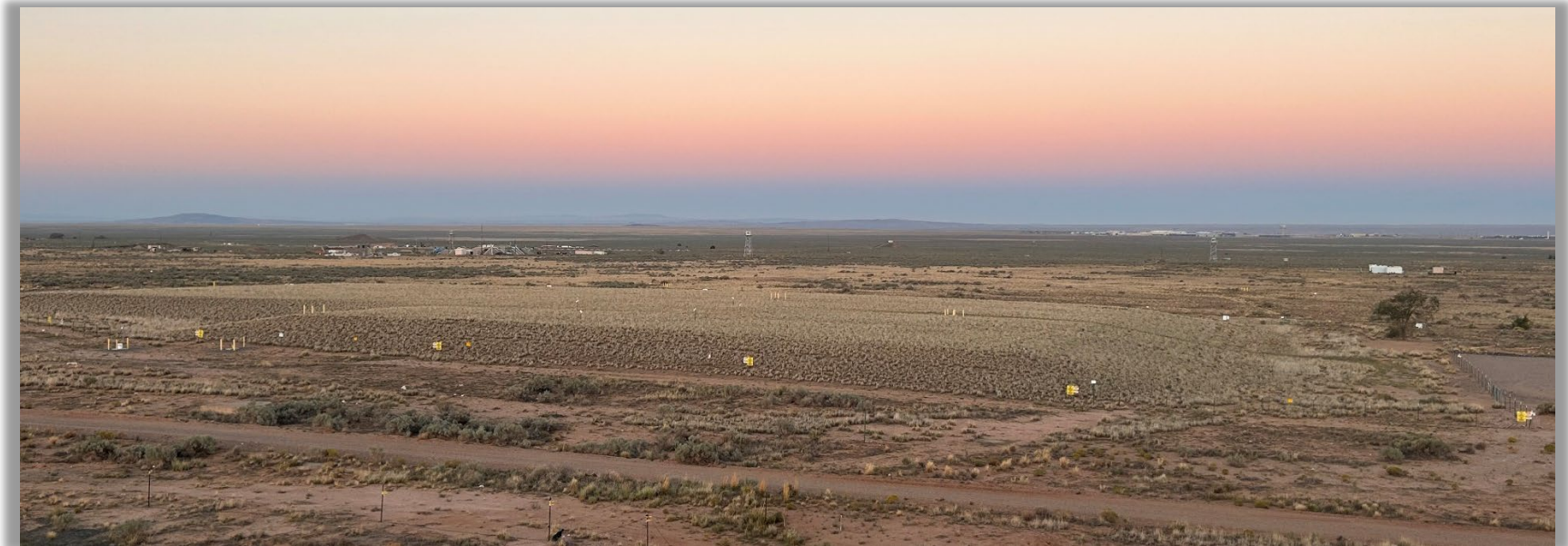
Figure 2-7 Mixed Waste Landfill Evapotranspirative Cover in September 2023 View Looking West
