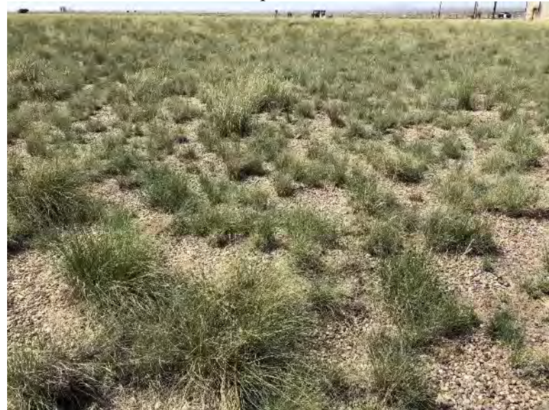
Northeast portion of the ET Cover
