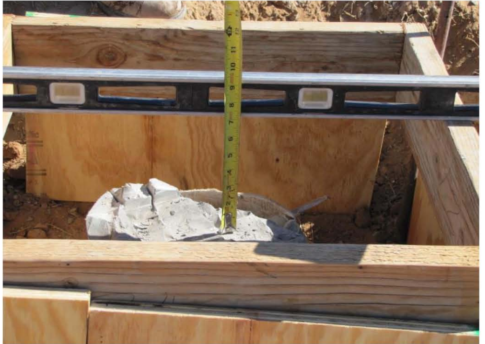
Repair of CWL-MW 2BU/L Concrete Pad February 2013
