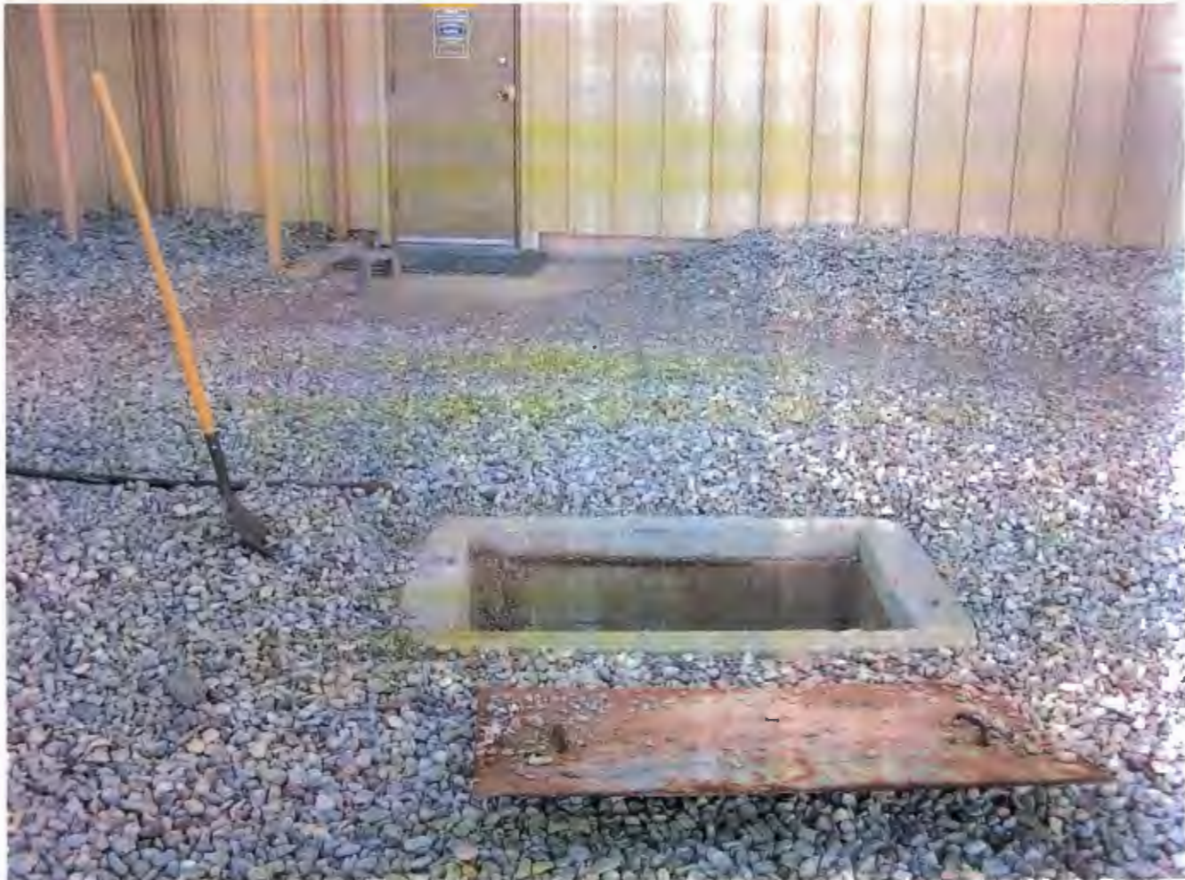
Photograph No. 3: Concrete Sump (looking south with B1079 in the background).
