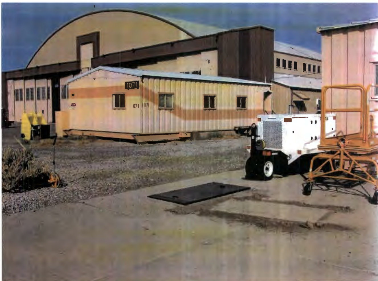
Photograph No. 1: Pipeline Valve Box Cover (looking Northwest with B1071 and B1079 in the background).
